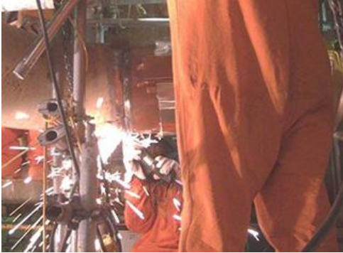
Grinding and cutting can disturb oxide layers in piping
