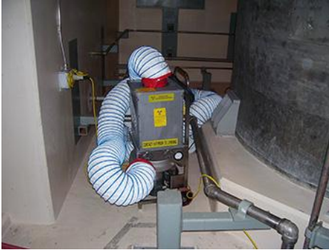
Hepa ventilation used as engineering work controls
